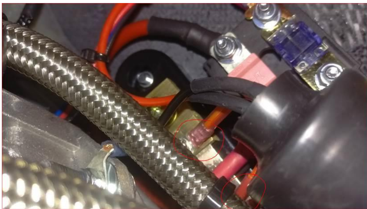
Fig 4: Shunt, new Installation
