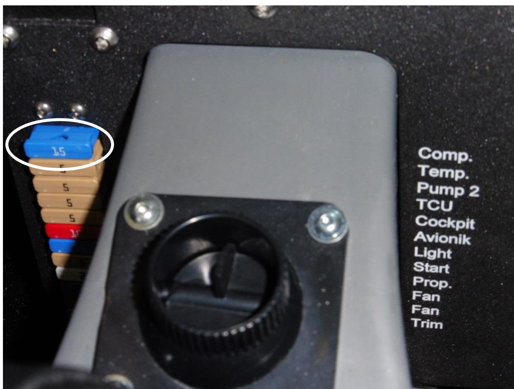
Fig. 2: 15A Fuse Compressor
